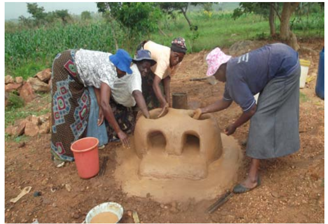
Firewood saving stove construction
